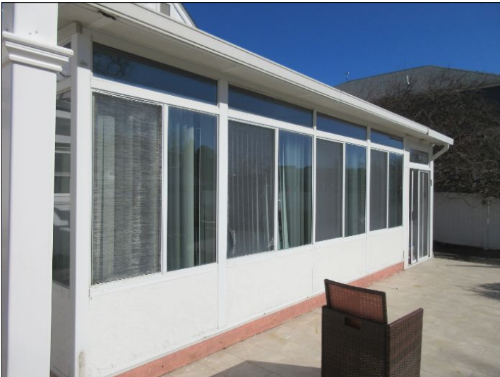
Rear sun room - Satisfactory
