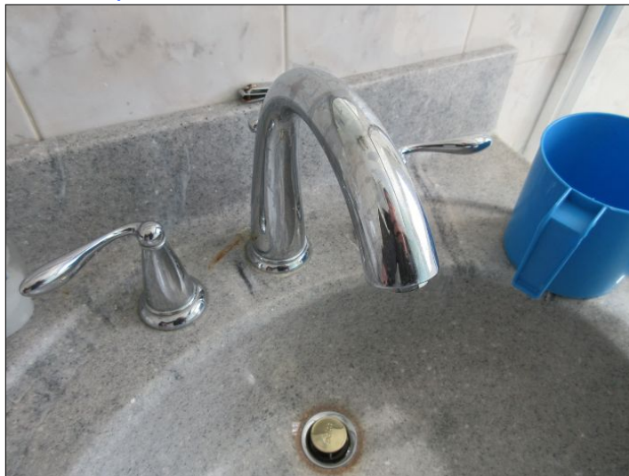
No deficiencies noted on the inspected faucets.
