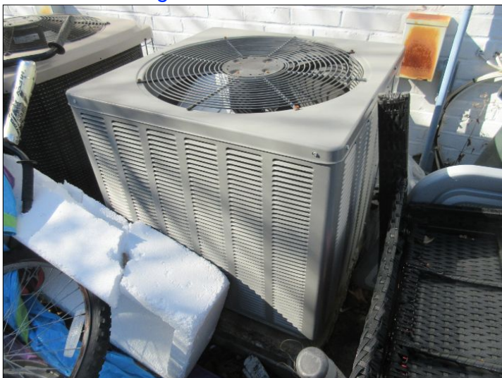
1st floor A/C system - 3 ton - Mfg 2013
