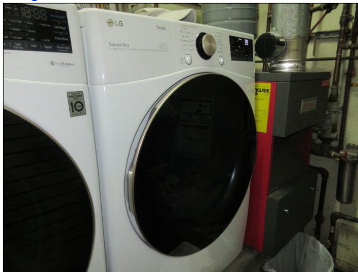
Operated as designed using normal controls
