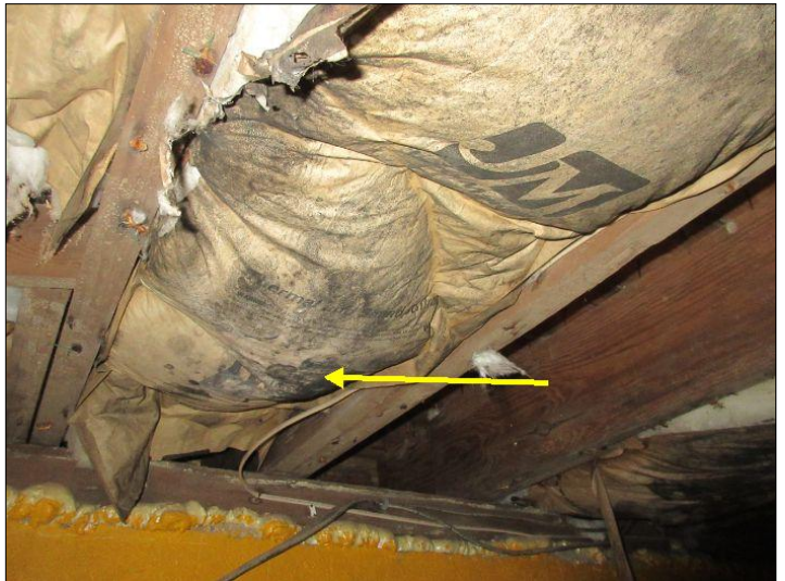
Mold-like bio growth observed. Professional testing & evaluation advised.
