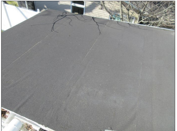
Roof appeared serviceable condition at time of inspection
