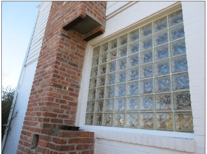
Appeared functional at time of inspection (Right side)
