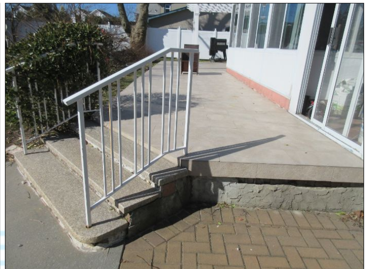
No deficiencies noted
