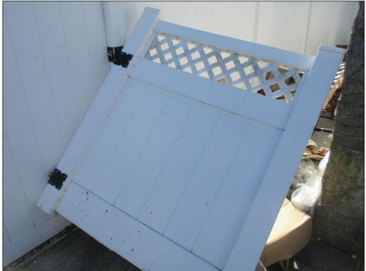
Damaged gate noted (Left of garage)
