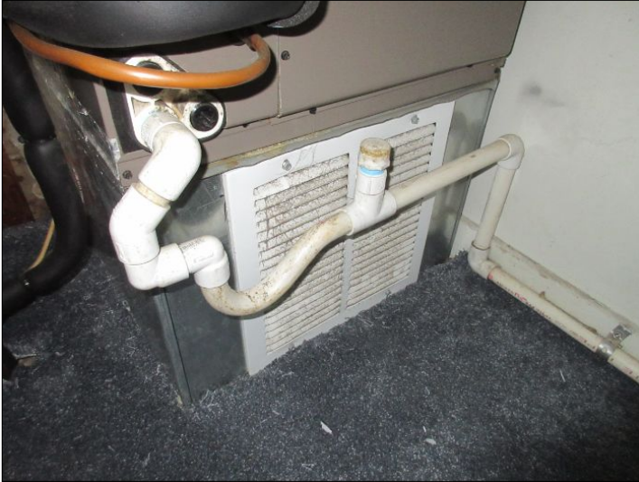
2nd floor - No deficiencies noted
