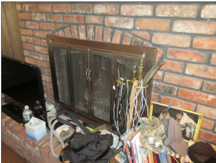
Appeared functional at time of inspection (Master Bedroom)
