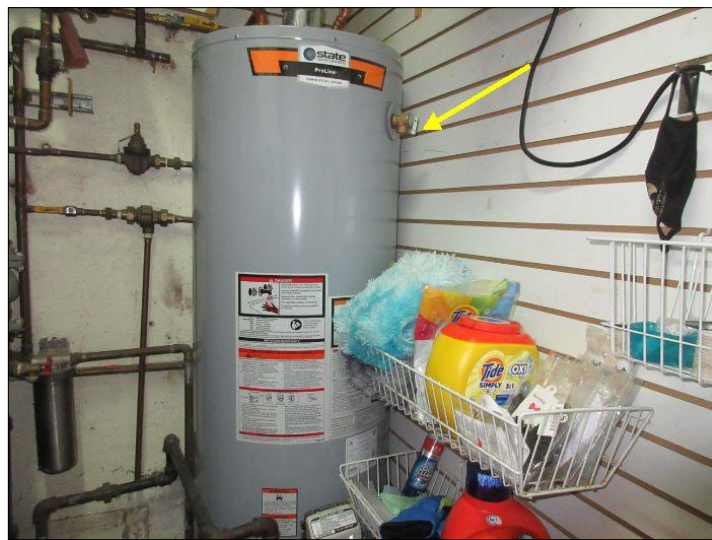
SAFETY: Temperature Pressure Relief (TPR) Valve extension pipe is missing
