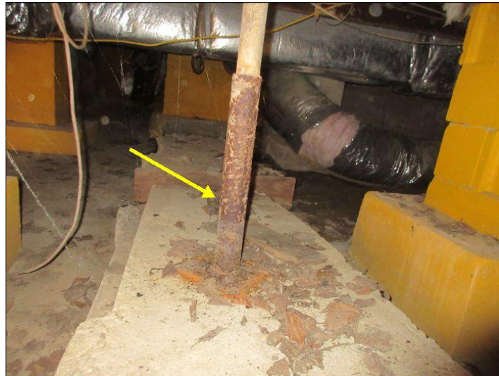
Temporary support column noted
