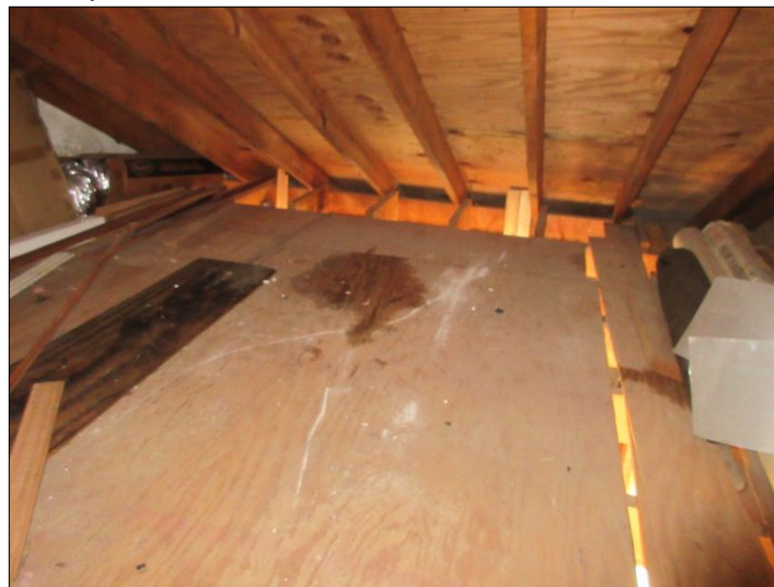
Rear area - Satisfactory
