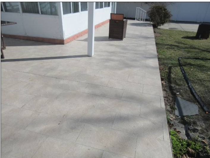
No deficiencies noted
