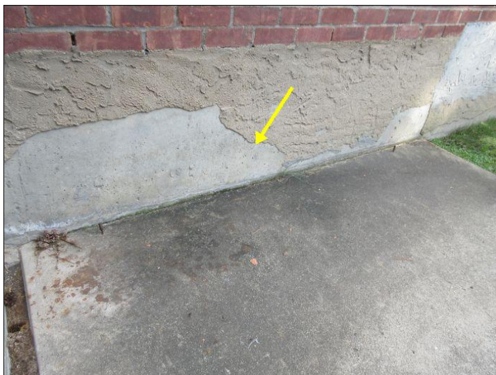
Damaged parking noted
