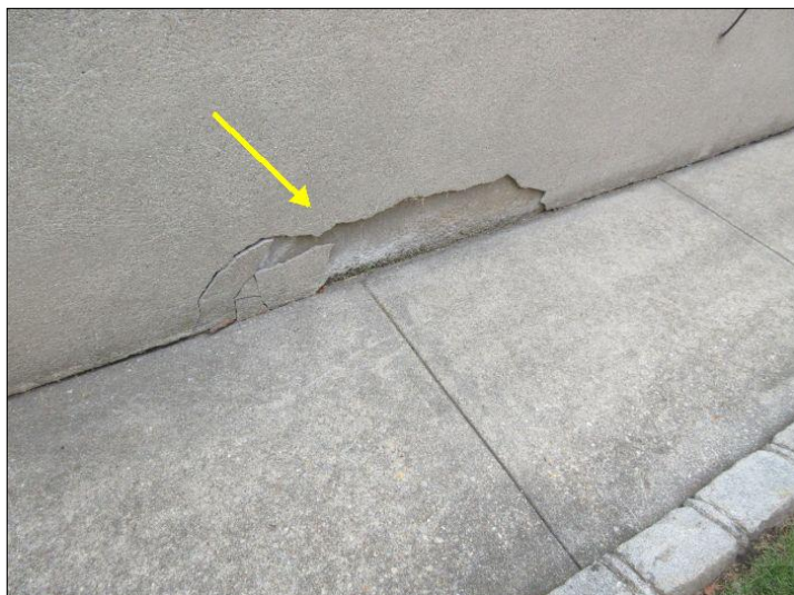
Damaged parking noted
