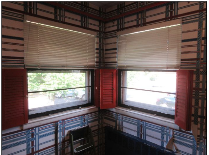
DEFERRED COST: Windows are original. Consider upgrading to double pane, thermally insulated, more efficient type.
