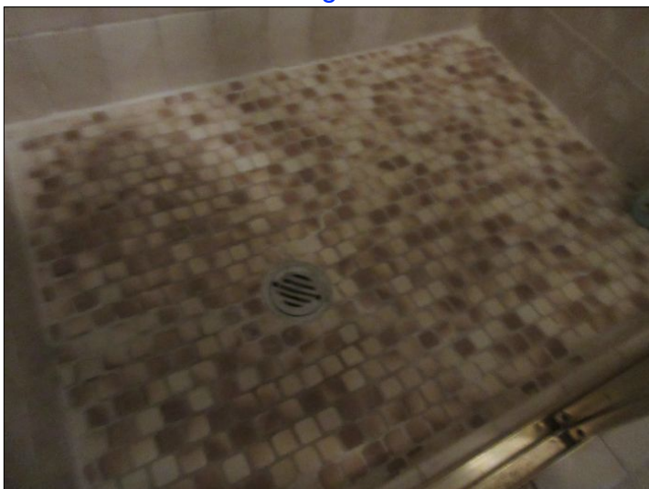
Appeared functional, at the time of inspection
