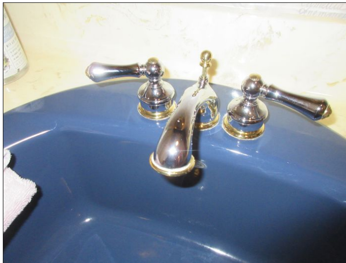
Left faucet - No deficiencies noted
