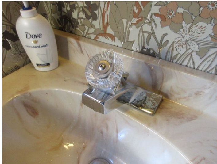
No deficiencies noted on the inspected faucets.
