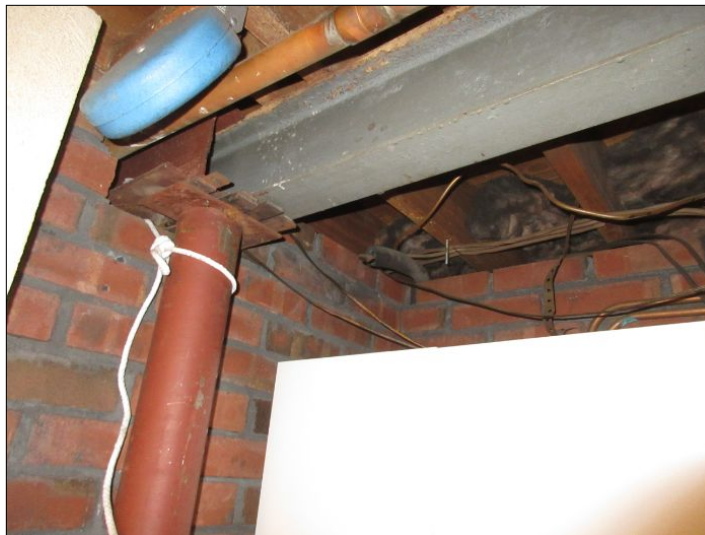
No deficiencies noted at the visible areas.
