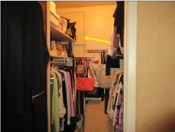
Access in Master Bedroom closet restricted due to personal belongings
