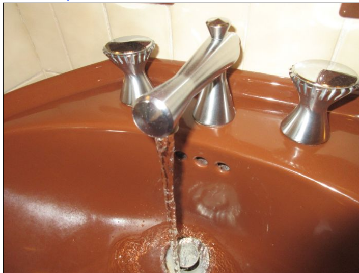
No deficiencies noted on the inspected faucets.
