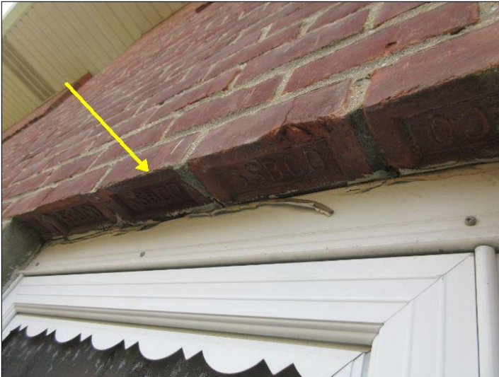
Missing lintel noted at doorway opening (Garage)
