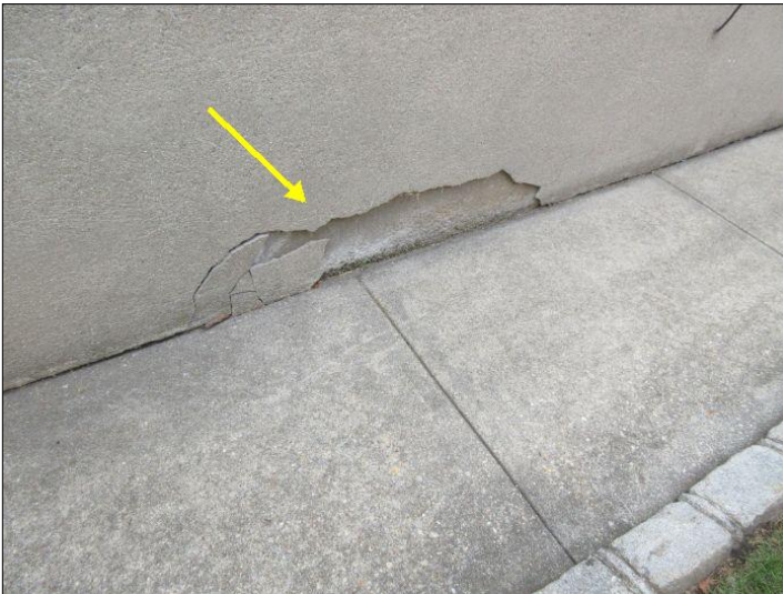
Damaged parging noted
