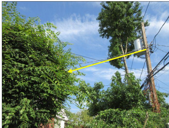
Sheathing on service entrance wires is in deteriorated condition. Recommend budgeting for upgrades to electrical service.
