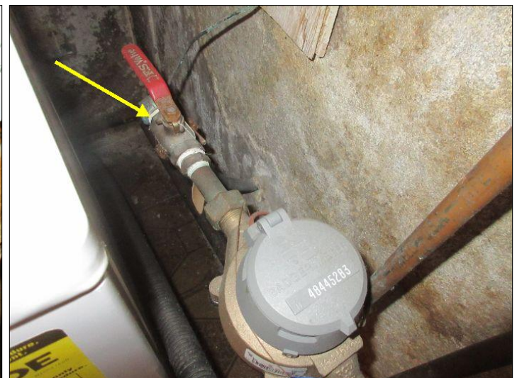
Main service shut off valve
