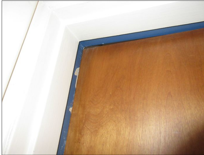
Door sticks, does not close, needs adjustment (Bedroom #3)
