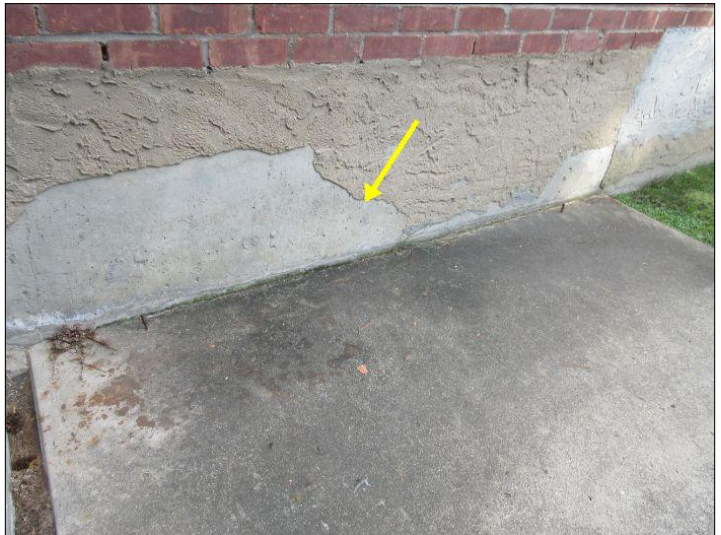
Damaged parging noted
