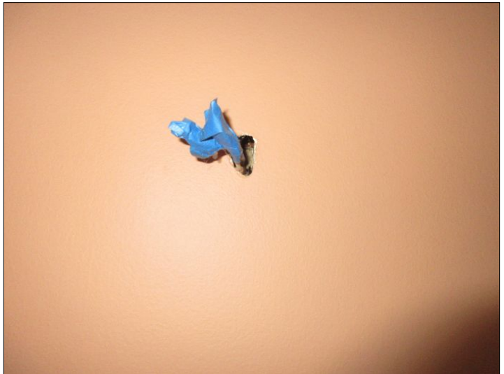
Exposed wiring noted from removed wall sconce. Recommend securing by licensed electrician (Living Room)
