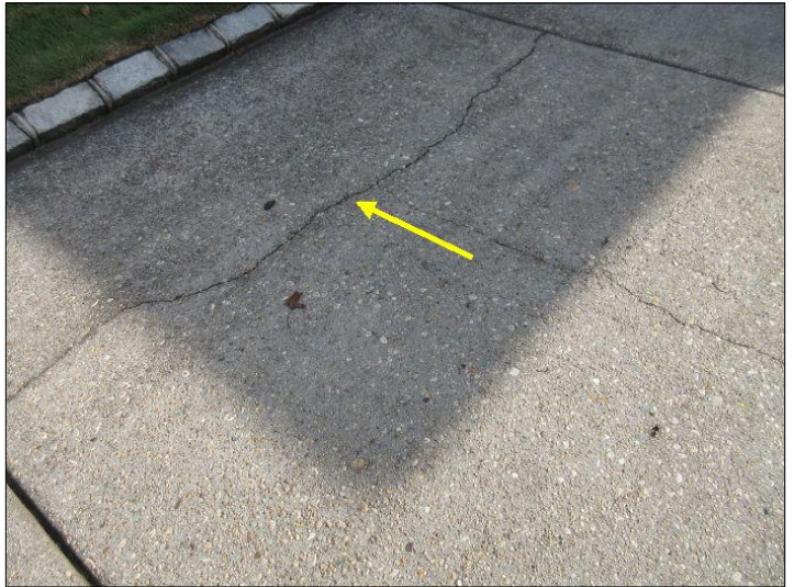
Common cracking noted
