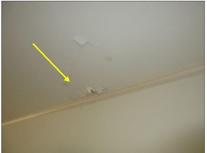
Blistering noted - Area did not appear wet when tested with moisture meter - Recommend monitoring (Living Room)
